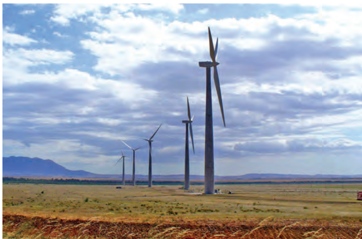
Aveg 135 MW wind power plant with 46 turbines.
